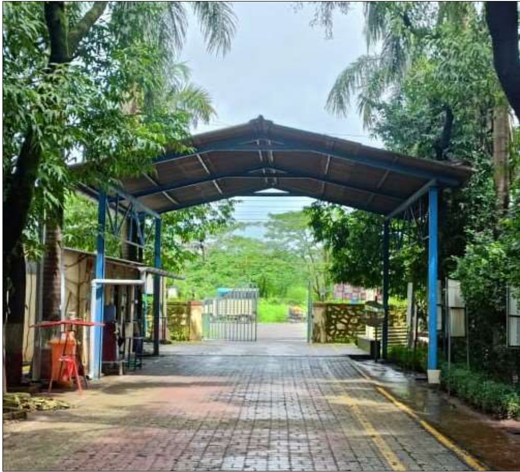
Shed work at Security Gate No.1
