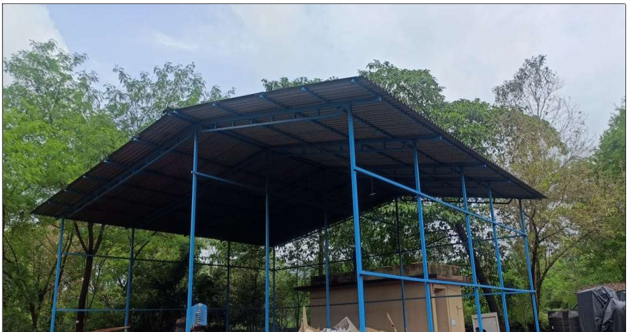
Shed Work at Scrap yard
