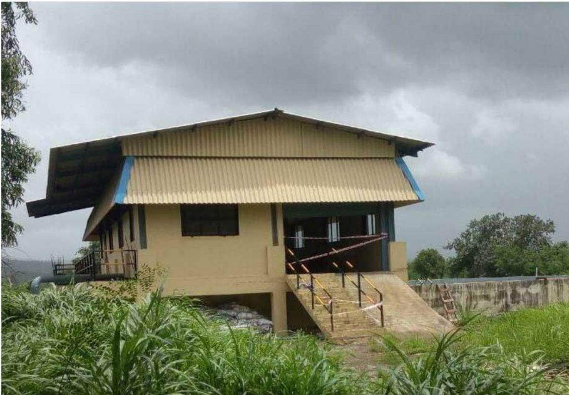
Construction of pump house above Low COD receiving sump.
