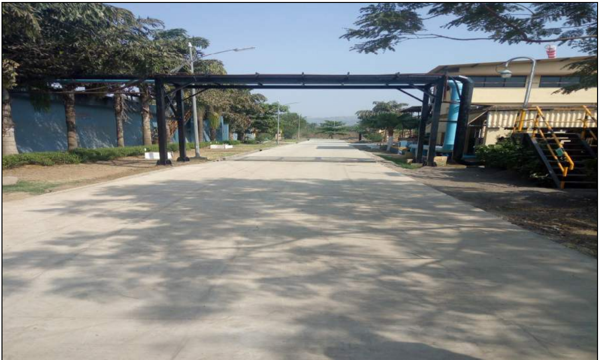
After Construction RCC Road
