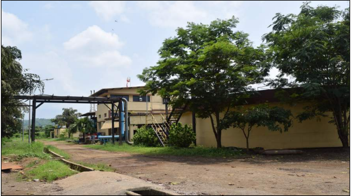
Before Construction RCC Road
